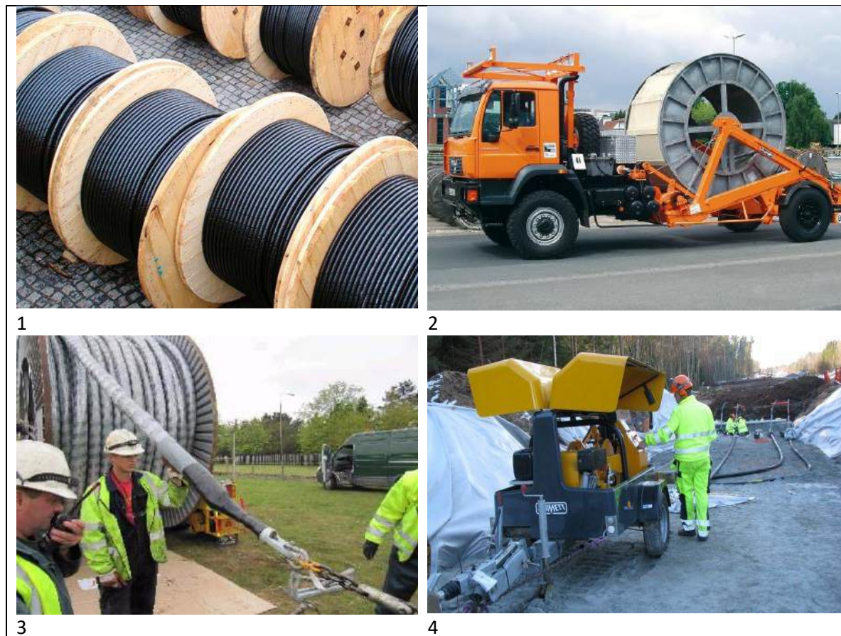
Figure 3.10. Examples of 220 kV cable drums (1), vehicles with a cable trailer (2), EHV cable winching operation (3), example of a cable winch (4) [source: okorder.com, lancier-cable.de, rampionoffshore.com, watucab.pl]
